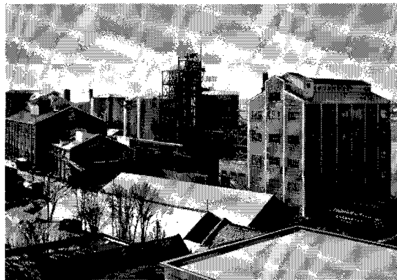
The Sandar Fabrikker fatty-acid-glycerine plant is located at Sandefjord, Norway—the whaling center of the world. Designed and built by Foster Wheeler, it is one of the largest specialty fatty acid processing plants in Europe, contributing substantially to the world's production of fractionally distilled fatty acid.
